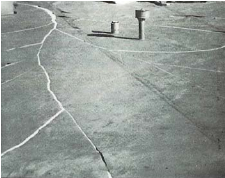
plasticizers are lost, PVC membranes will embrittle and be susceptible to attering even by foot traffic.
